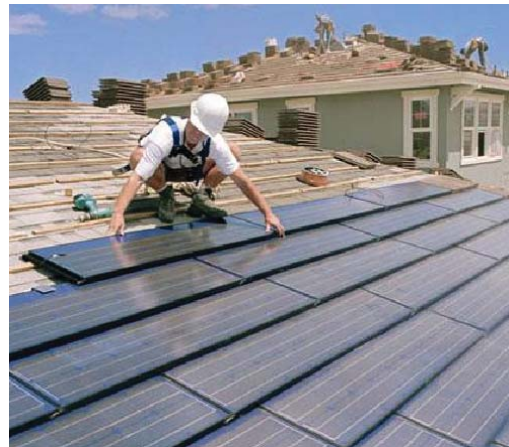
Photovoltaic panel installation on a residence
