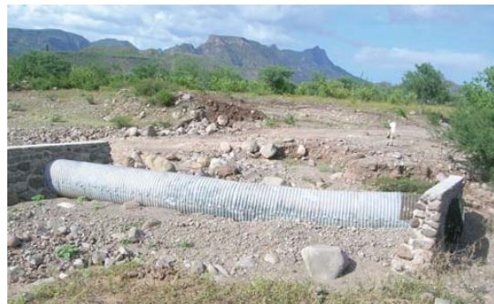
Disturbed Drainage Culvert outside of Loreto
